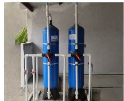
50 KLD for M S Homes Constructions
