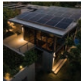
Solar Home Power
