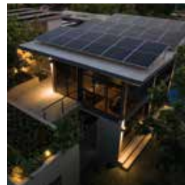
Solar Home Power
